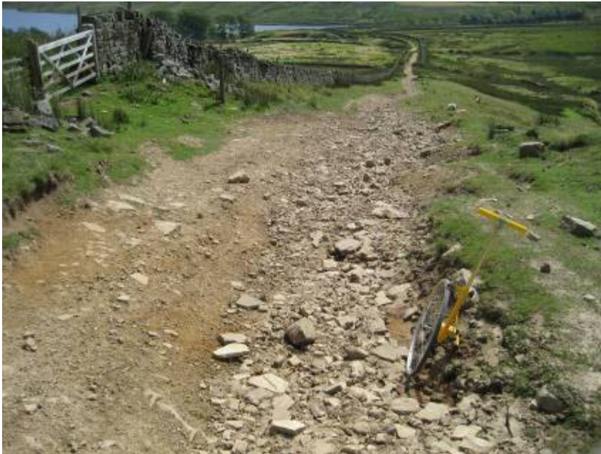
NYCC July 2007, section between zig zags and Lodge
